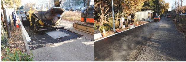
(l) Paving of surface course (m) Finished pavement Fig.5 Flow of coil burial work
