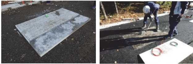
(a) Soil retaining board (b) Soil-retaining board after burial
