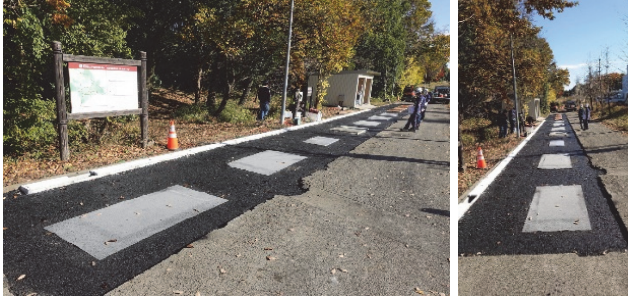
(k) Complete coil installation and wiring using the four methods
