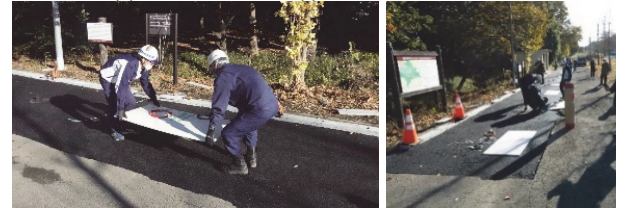
(g) Coil installation 1 (h) Coil installation 2
