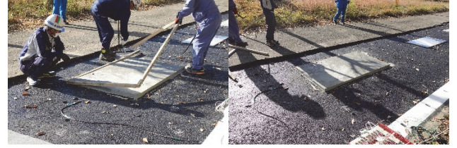
(c) Removal of formwork. (d) Finished Fig.9 Case 4: Grout material, cement for pouring
