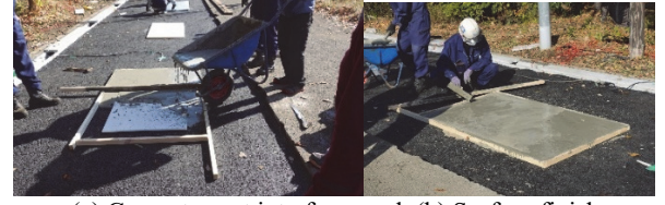
(a) Cement grout into formwork (b) Surface finish
