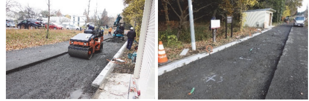
(c) Base course (MSCS) (d) Piping setup
