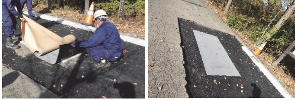
(a) Laying of RC mesh (b) Finished RC mesh Fig.6 Case 1: RC mesh
