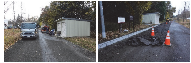
(a) Cutting (b) Removal of asphalt mixture
